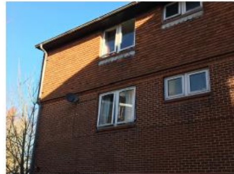
Courtyard materials and treatment.
