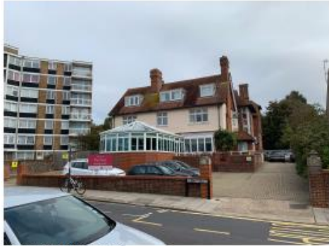
Main frontage to Furze Hill.
